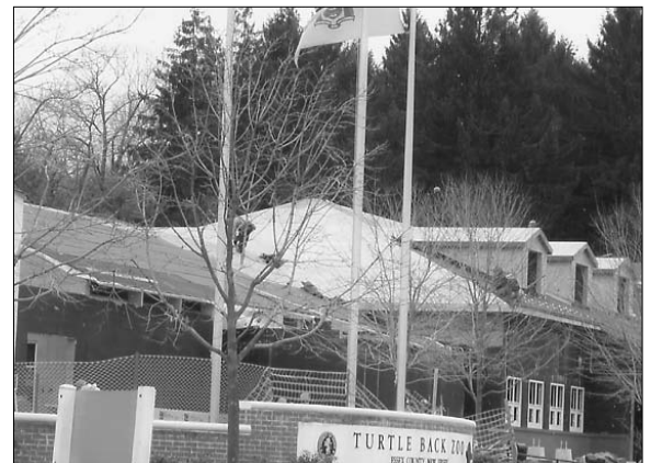
The Reptile House and Education Center under construction
